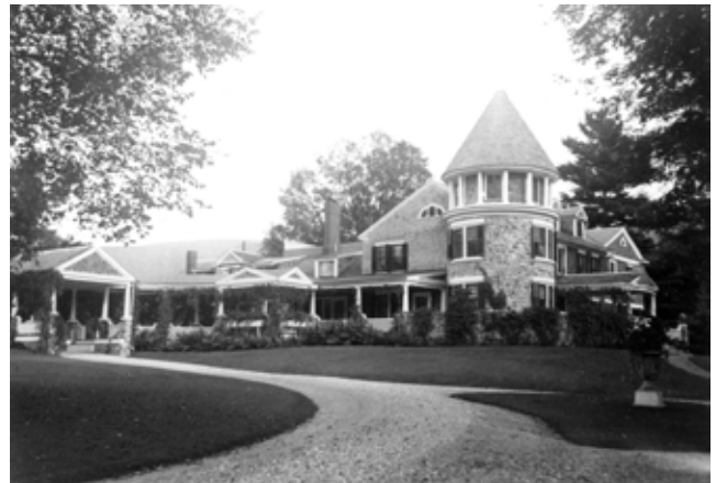
The Cascades, on River Road, home of U.S. Minister to Hungary (1933-1941) under President Franklin D. Roosevelt, John F. Montgomery from 1919-1954. Image a gift of Mr. Montgomery's grandchildren.
